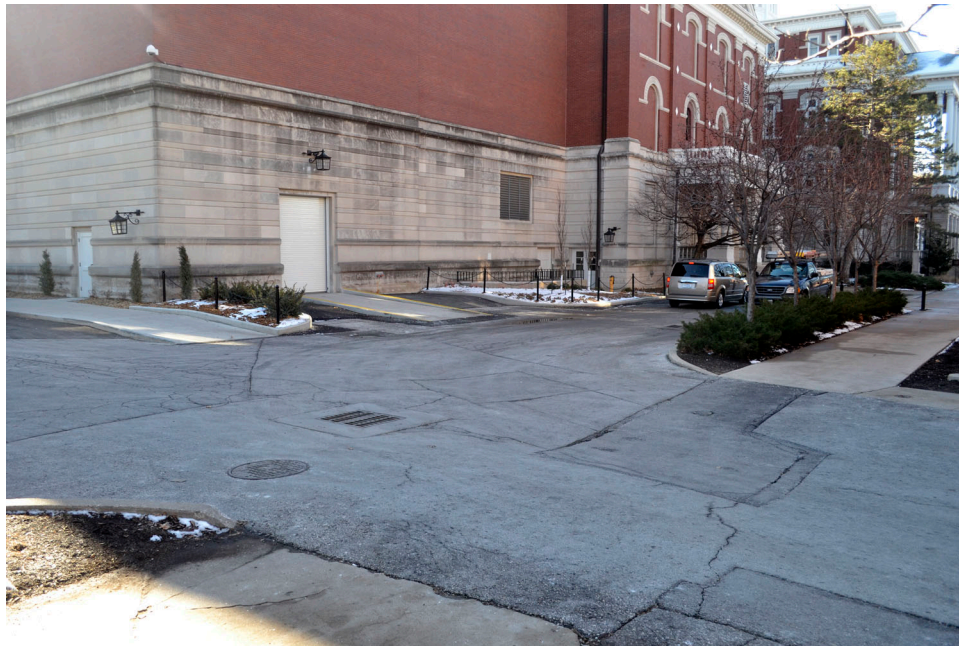
View of the loading area outside the Load Door
