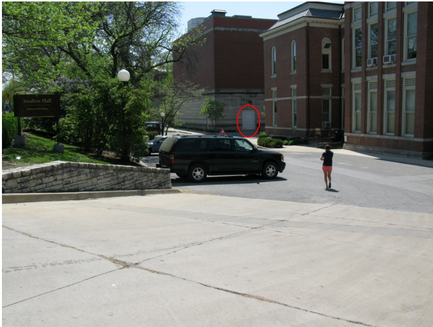
View of the loading door from the street
